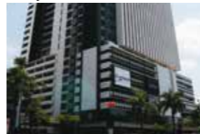
Malaysia Plaza 33 Office Block A
